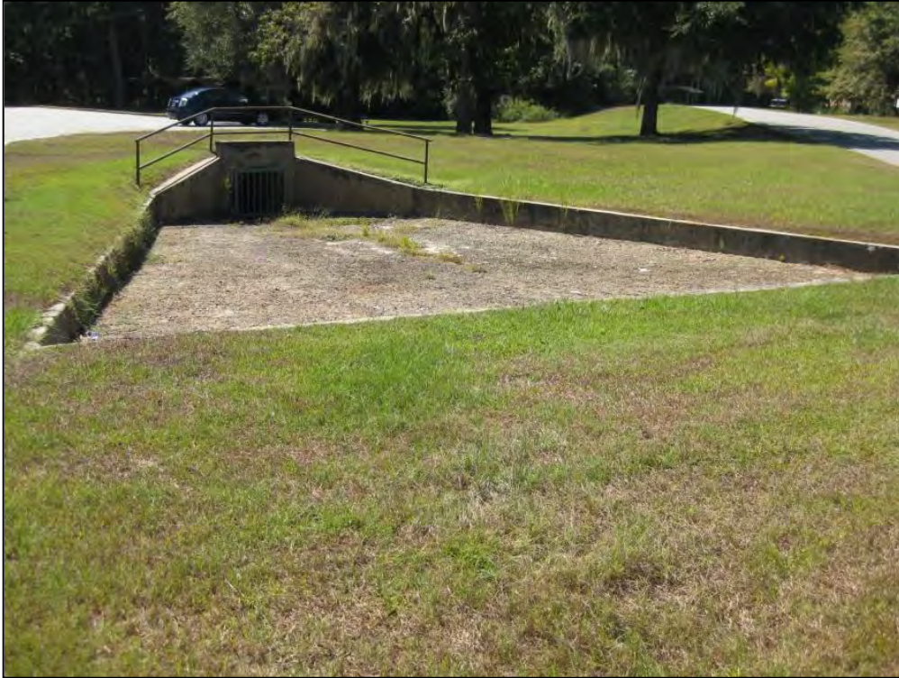
Figure 35. Facility 1704, Spillway at Mission Lake, facing south.
