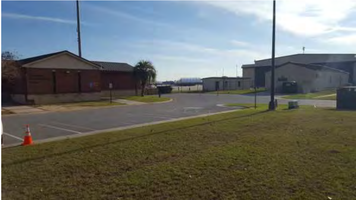
Image 9: View South of Structure 618, facing south
