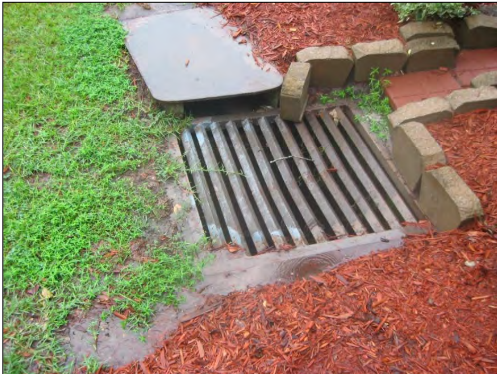
Figure 48. Facility 20202, Storm Drain, detail view of inlet.
