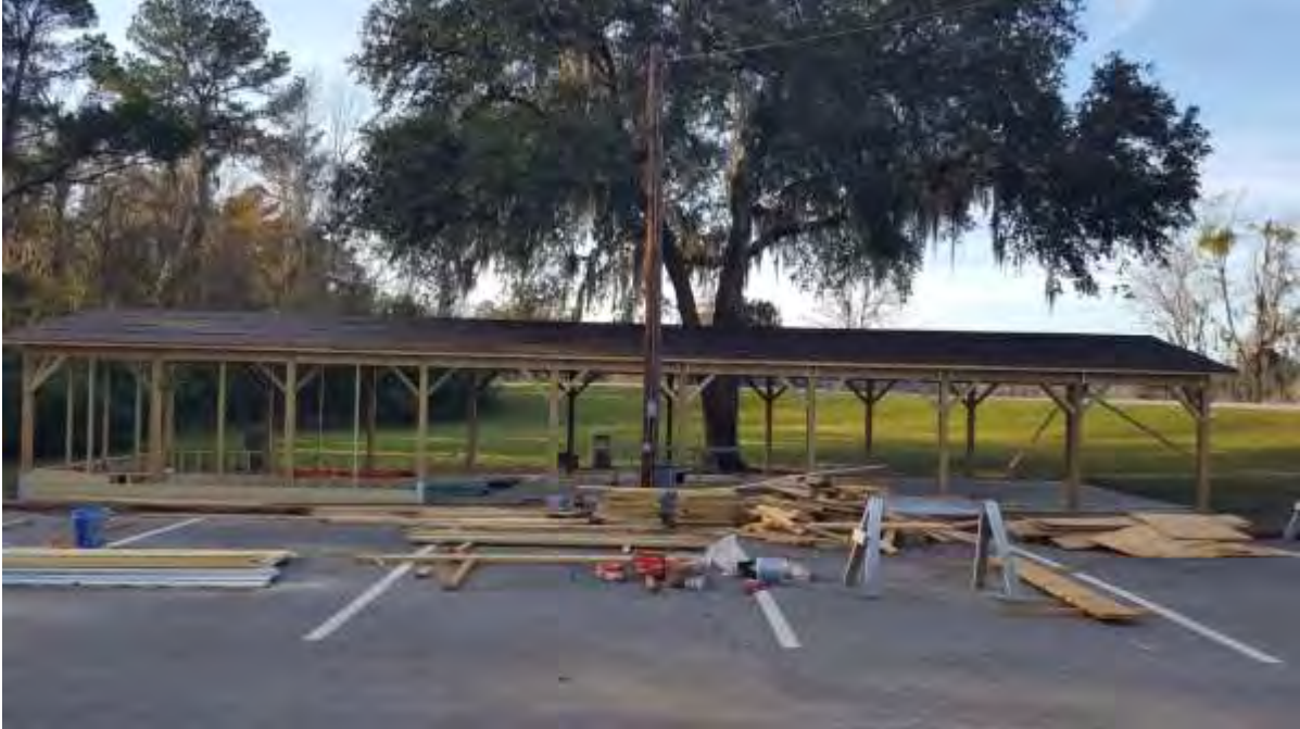
Image 13: Facility 7001, Non-Historic Wood Pavilion, facing northwest
