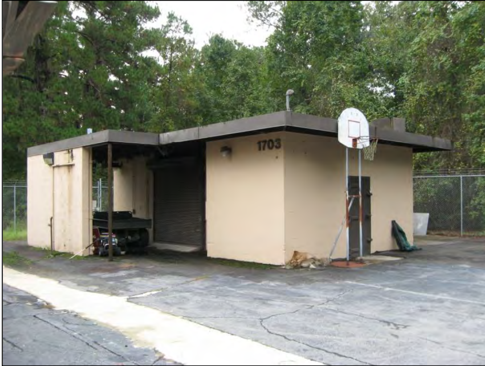
Figure 34. Facility 1703, CE Storage building, facing southeast.
