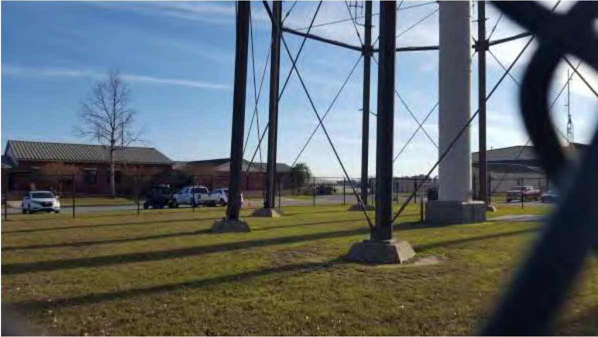
Image 8: View North of Structure 618, facing south
