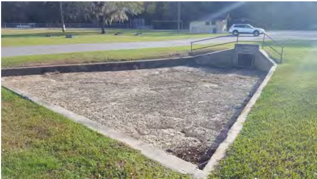
Image 16: Facility 1704, facing southwest
