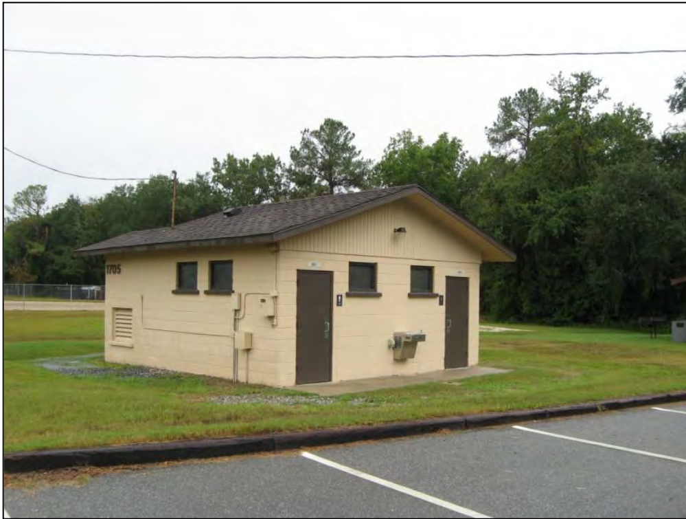
Figure 36. Facility 1705, Latrine Facility at Mission Lake, facing southeast.
