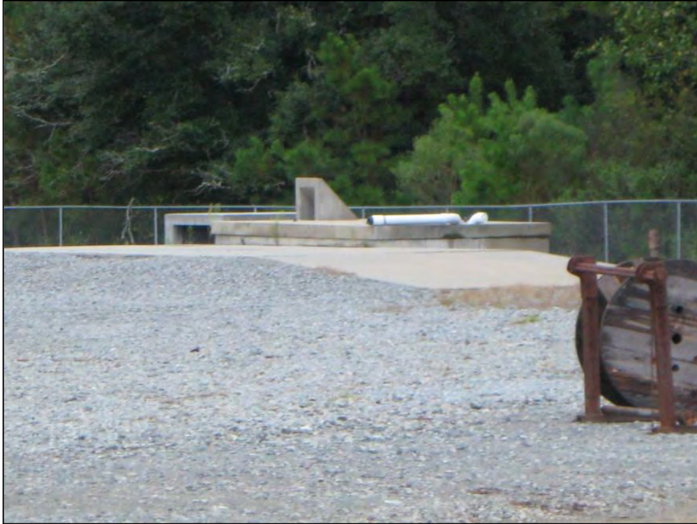
Figure 40. Facility 3148, CEF Storage structure, facing east.
