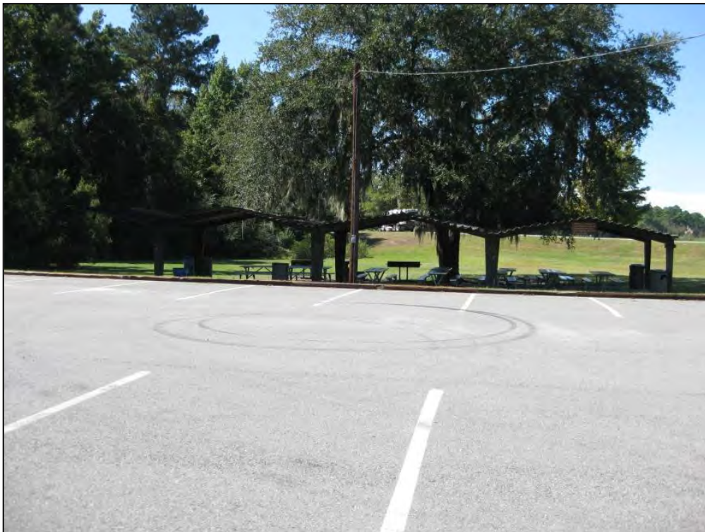
Figure 44. Facility 7001d, Metal Pavilion, facing west.
